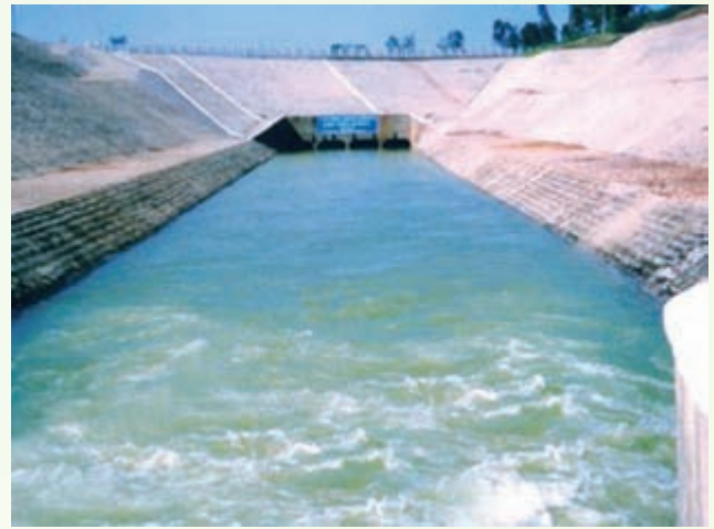
Chennai Water Project
